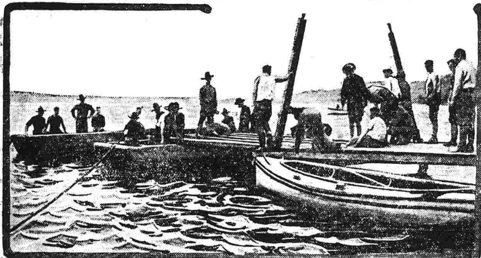
The young engineering officers whom the government is training at the camp at Belvoir, Va., get not only theory, but actual practice in engineering problems. They are seen here constructing a light pontoon bridge.
